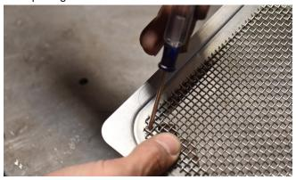
5. It will only require slight working of the mesh to enable the screw to pass through. When ready, pass the stainless steel button head cap screw first through the screw hole in the Inner Fender, then through the just-rounded opening in the Mesh Insert.
